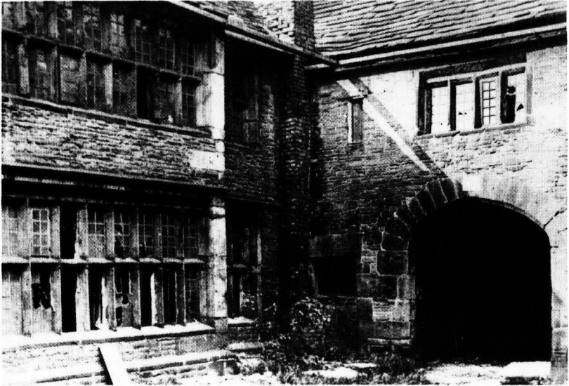
Belfield Hall: A corner of the courtyard showing its derelict state shortly before demolition c. 1914. (Manchester Public Libraries).
